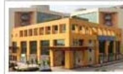
Hyderabad, Andhra Pradesh, India
